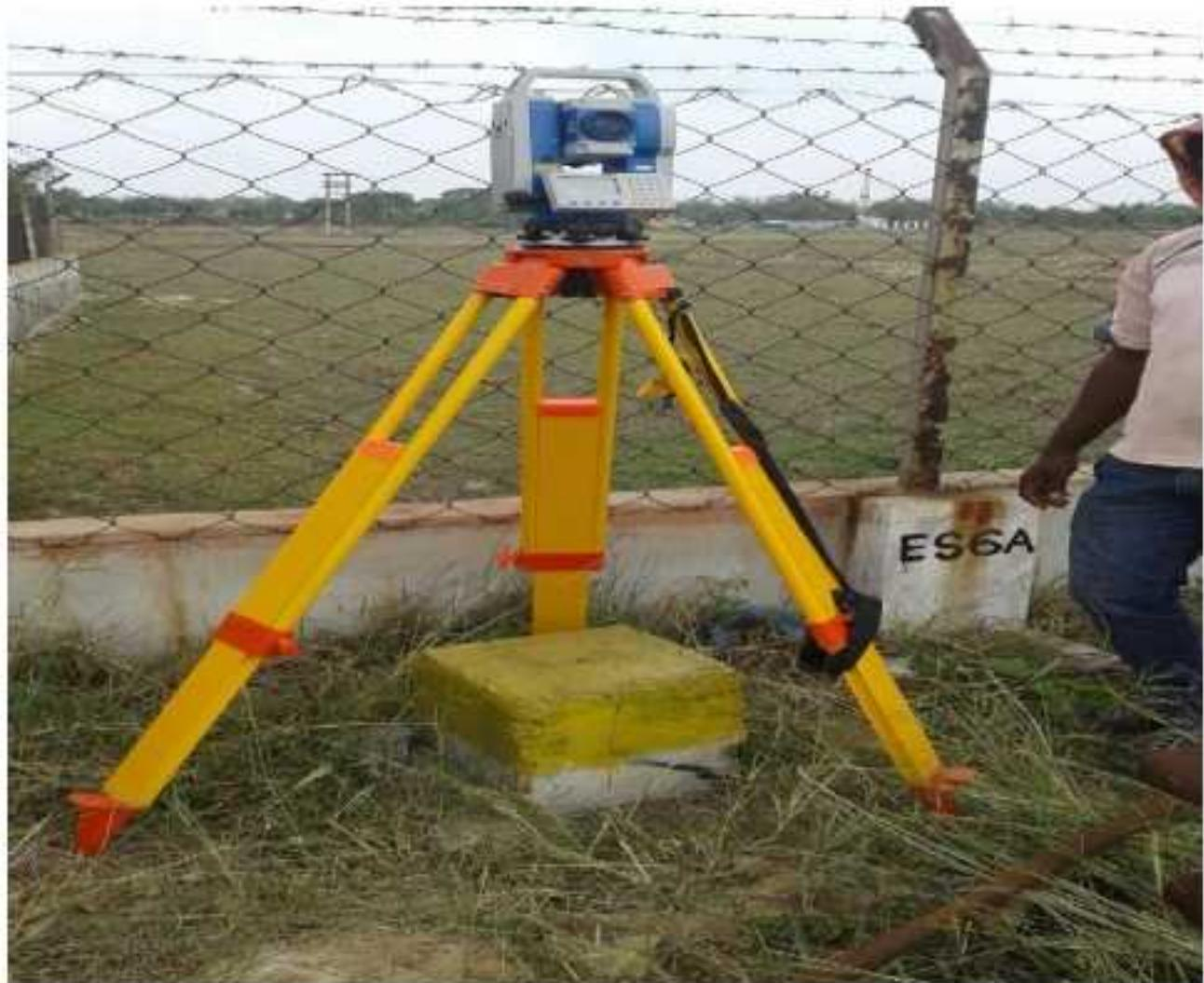
**Plate 2:** Subsidence monitoring station being established at ES 6A
